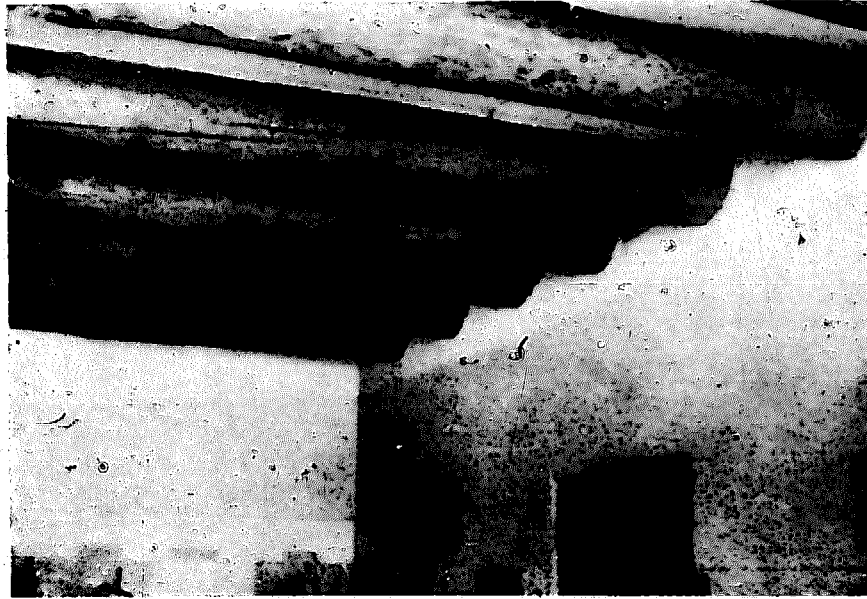
Figure 86. The large and small ends of the ceiling timbers (vigas) are alternated to provide a balanced appearance.
