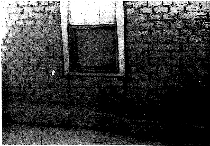
Figure 66. An overhanging window sill channelizes the rain into two rivulets, easily eroding the unprotected, nonstabilized wall surface.
