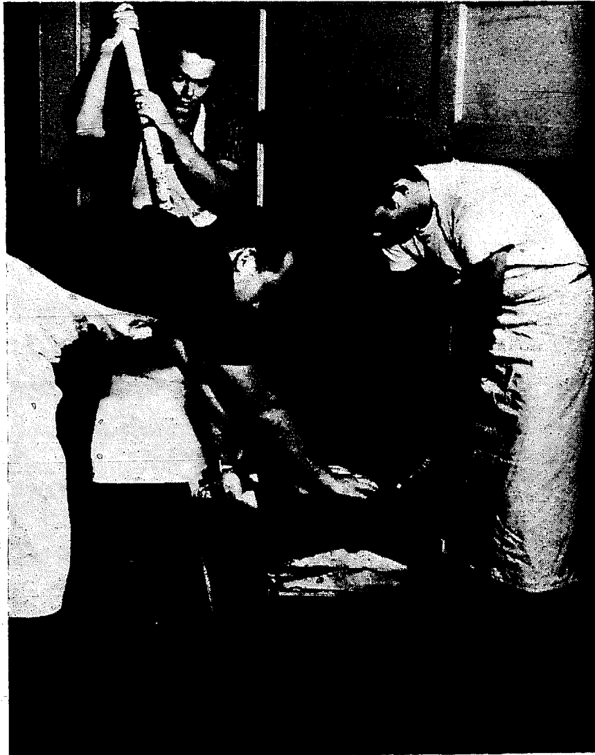
Figure 54. Charging mold box with soil mix.
